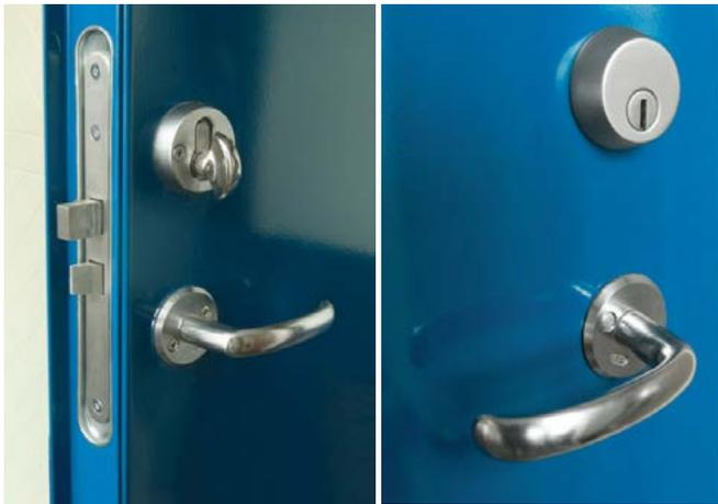
*Fire escape doors:* Alternatively, the doors can be fitted with 3 point heavy duty panic escape hardware to offer means of escape, which is accepted by the Secure by Design scheme.
